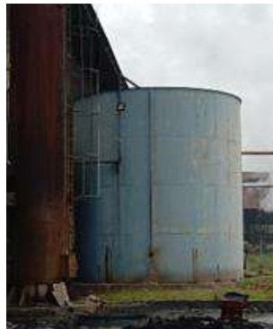
Gambar 3. 48 Feed Water Tank
