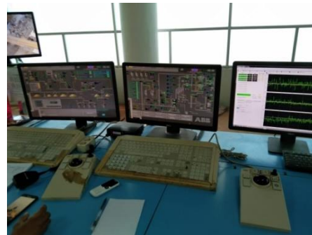
Gambar 3.26 Operator station CCR di PT. Semen Bosowa Maros
