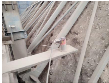
Gambar 3.2 Sensor Proximity Switch
