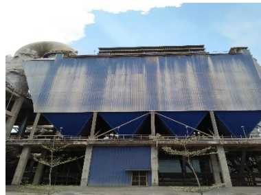
Gambar 2.6 EP (Electrostatic Presipitator)
