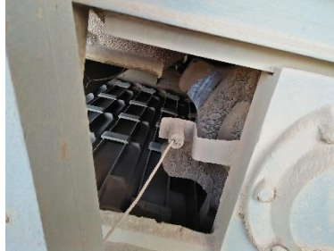
Gambar 3.8 Sensor Speed Switch
