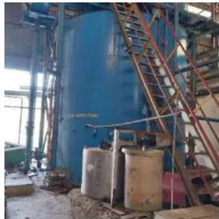
Gambar 3. 38 Feed Water Tank
