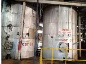
Gambar 3. 14 *Continuous Settling Tank (CST)*
